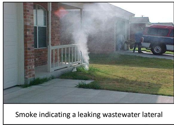
Smoke indicating a leaking wastewater lateral
